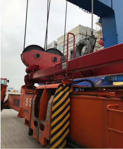
Fig. 2. Demonstration of the Data Acquisition sensory hardware placement on the crane spreader.
